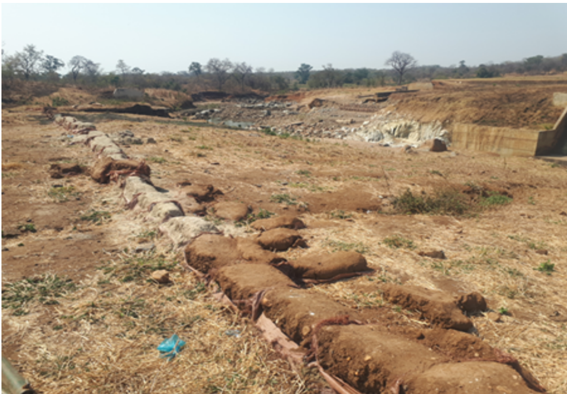
Plate 20: Sand bags installed to prevent further erosion of the spillway outflow channel
