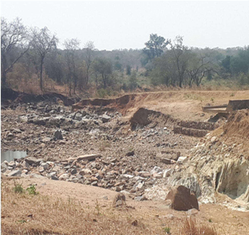
Plate 17: Erosion on the left bank of the training wall
