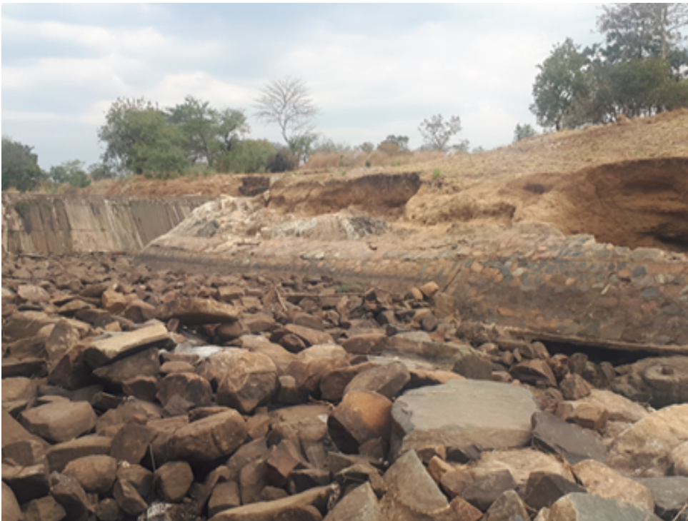
Plate 16: Erosion on the left bank of the spillway channel (both pictures showing this condition)
