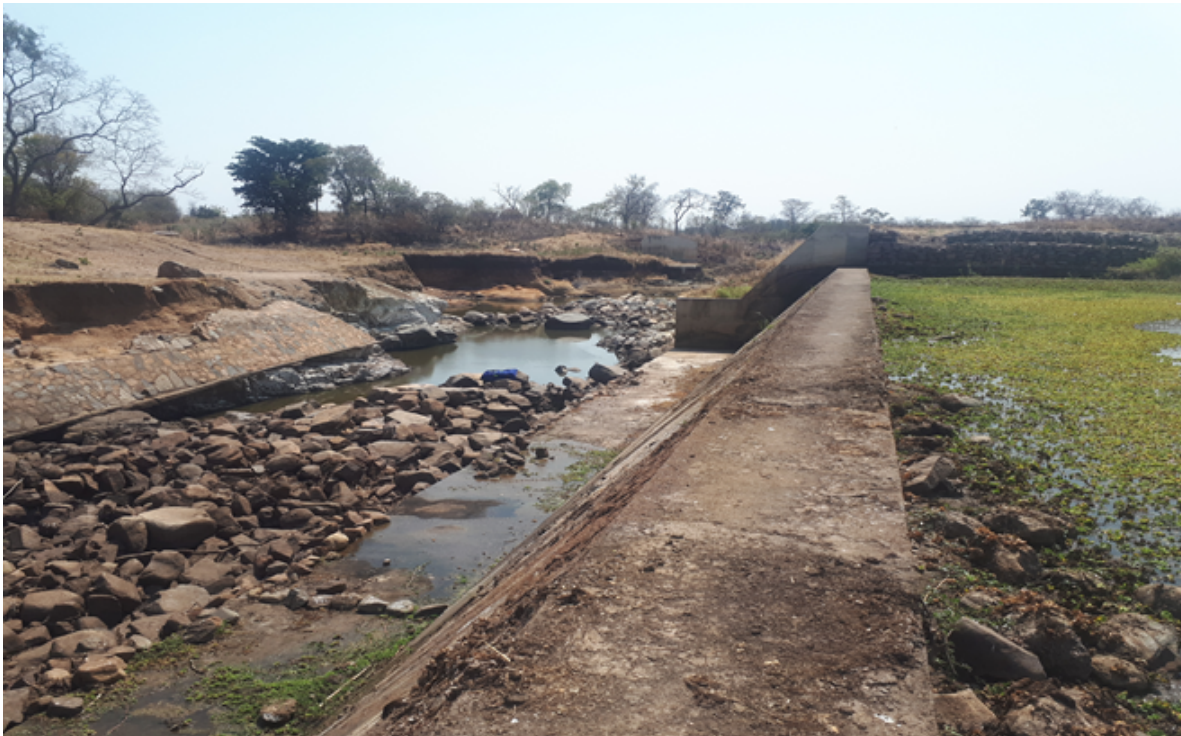
Plate 19: Eroded side of the spillway outflow channel
