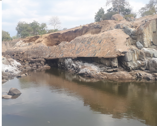
Erosion on the left bank of the spillway channel
