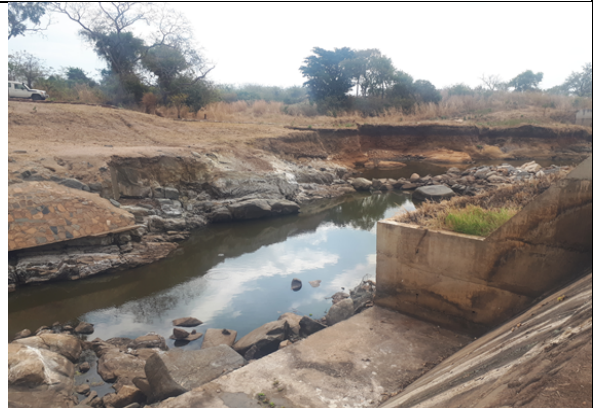
Eroded left bank of the spillway channel
