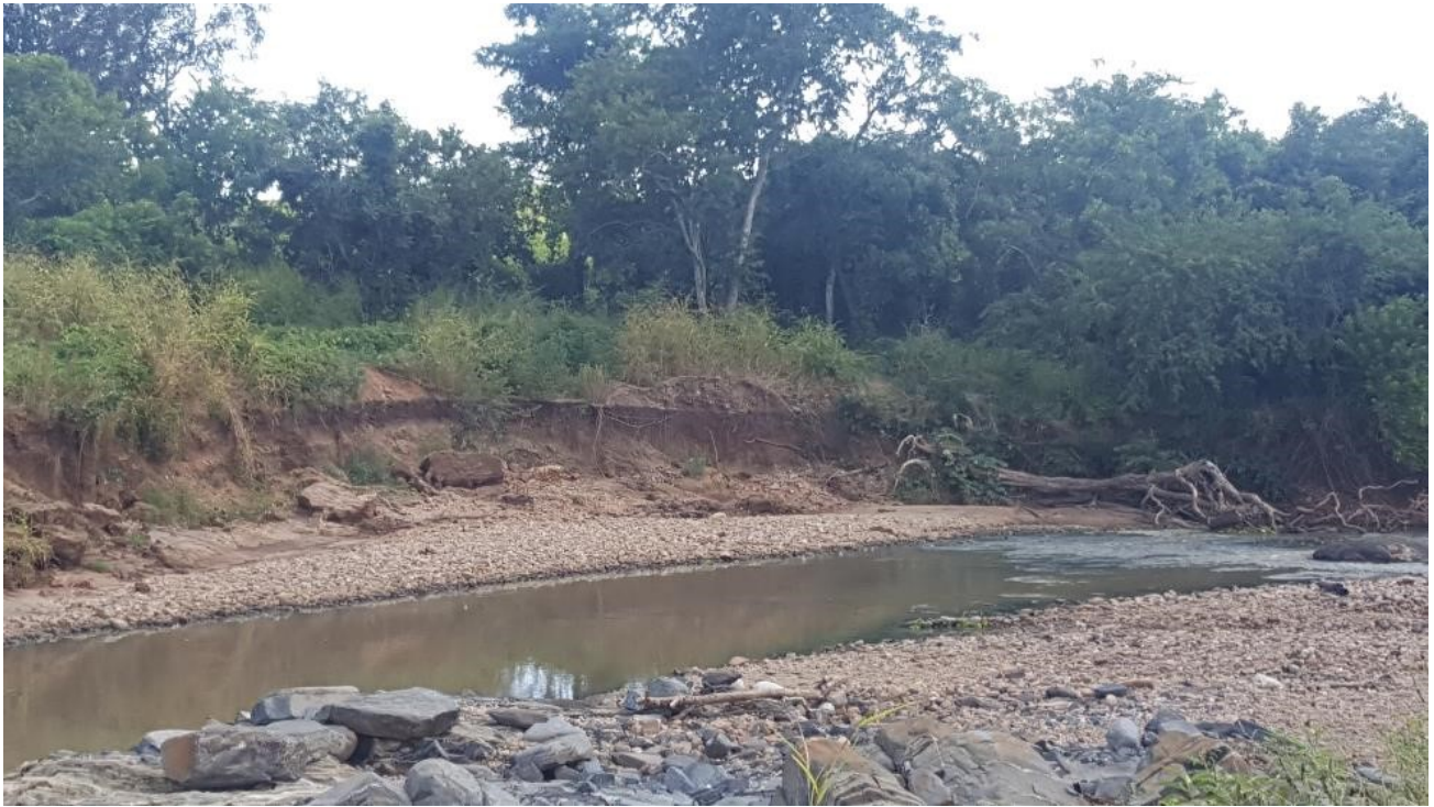
Plate 1: Chikowa Dam – Downstream showing exposed areas as a result of poor spillway conditions
