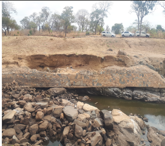
Eroded left bank of the spillway channel
