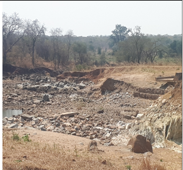
Eroded left bank training wall
