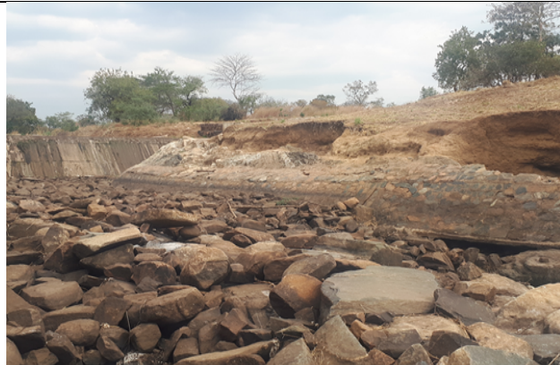
Heavily eroded left bank of the spillway channel
