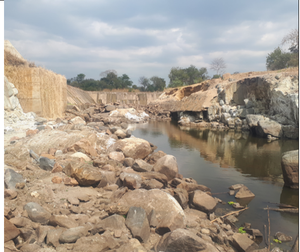
Eroded left bank of the spillway channel
