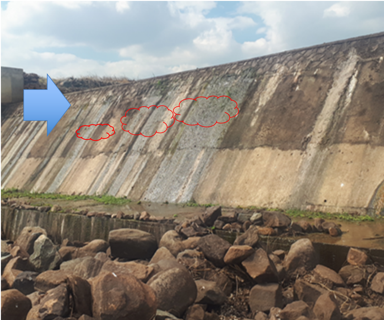
Plate 14: Seepage in-between the masonry crest and the concrete structure of the spillway
